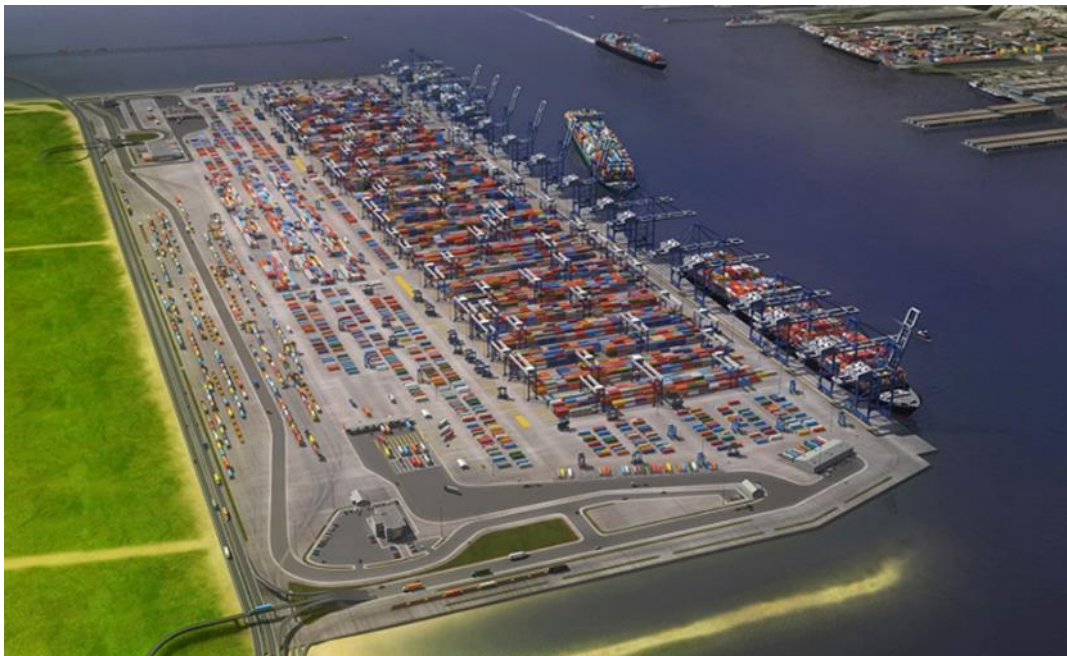
The future Craney Island Eastward Expansion Marine Terminal
